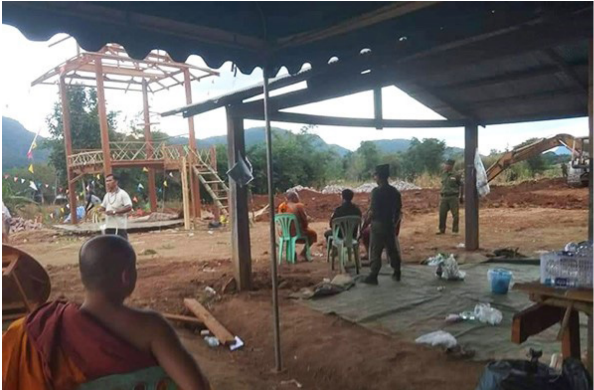
UWSA soldiers clearing stupa construction in Mong Ton, Dec 2018
