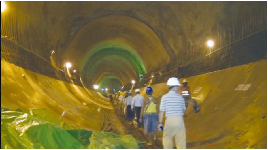
Water diversion tunnel of Upper Yeywa dam
