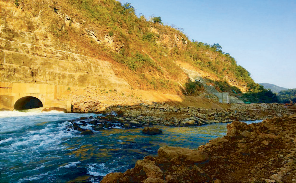
Upper Yeywa dam construction site
