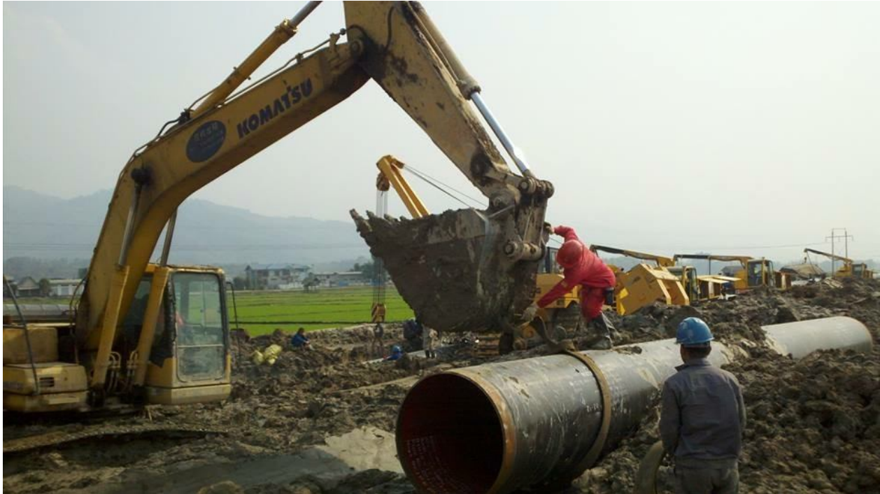
Oil and gas pipelines being laid in N. Shan State in 2012
