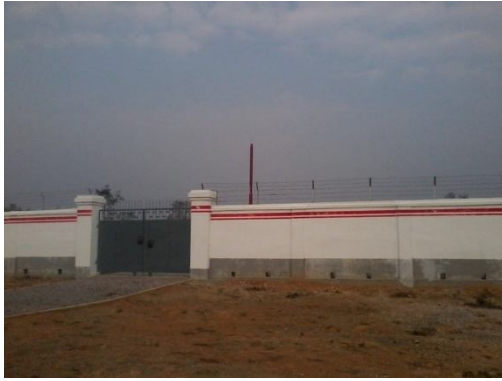
Pipeline pumping station near Nawng Arng
