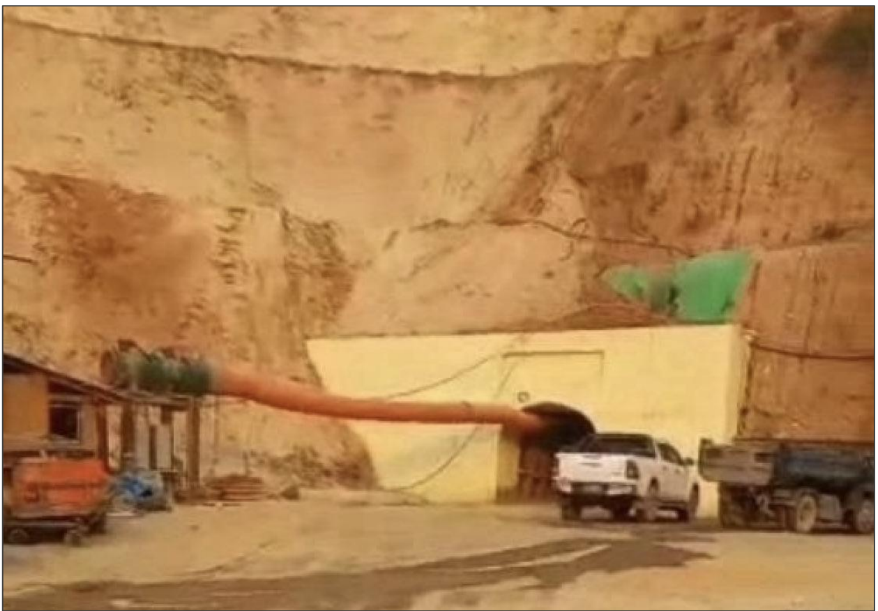
Tunnel at the Mong Jawd tungsten mine
