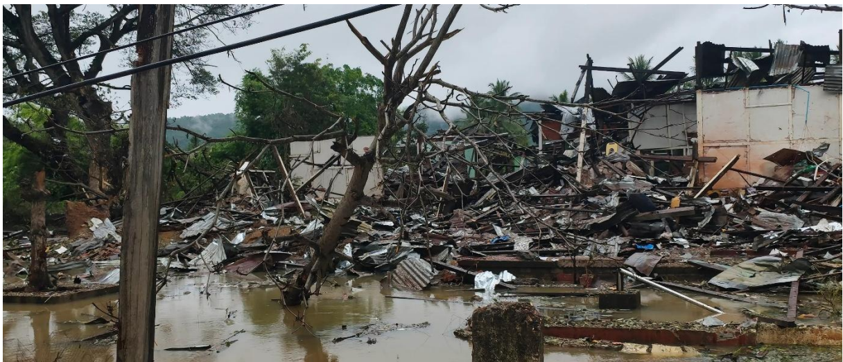
Hospital buildings in Ward 3, Mabein town, northern Shan State destroyed by SAC airstrike
